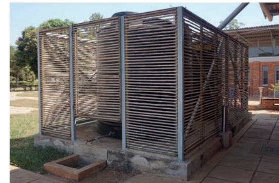
NTC Kaliro Two large plastic tanks at the end of each of the buildings are screened with bamboo to protect them from sunlight
