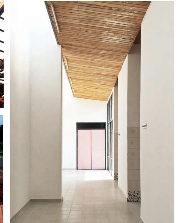
Rugerero Health Centre Umusave wooden planks with damp proof and insect preservative have been used as a ceiling material
