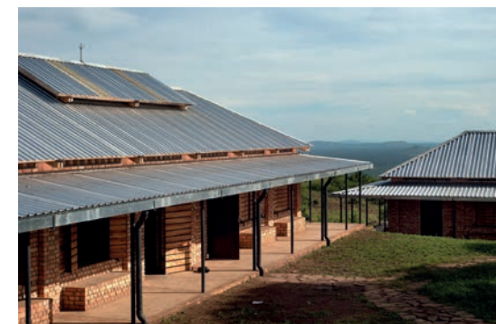
COF Primaries use silver reflective roofing to limit the thermal transfer of solar radiation to the classrooms spaces below
