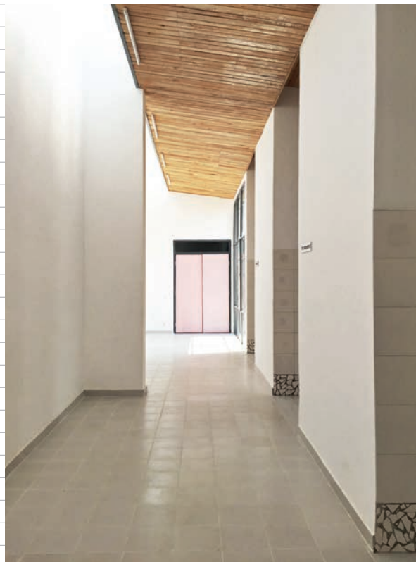
UMUSAVE WOODEN PLANK CEILING
