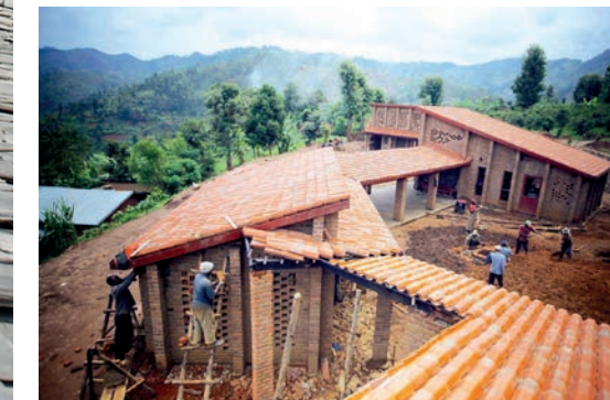
ECD&F Centres The fired clay tiles are a sustainable and locally sourced roof covering system
