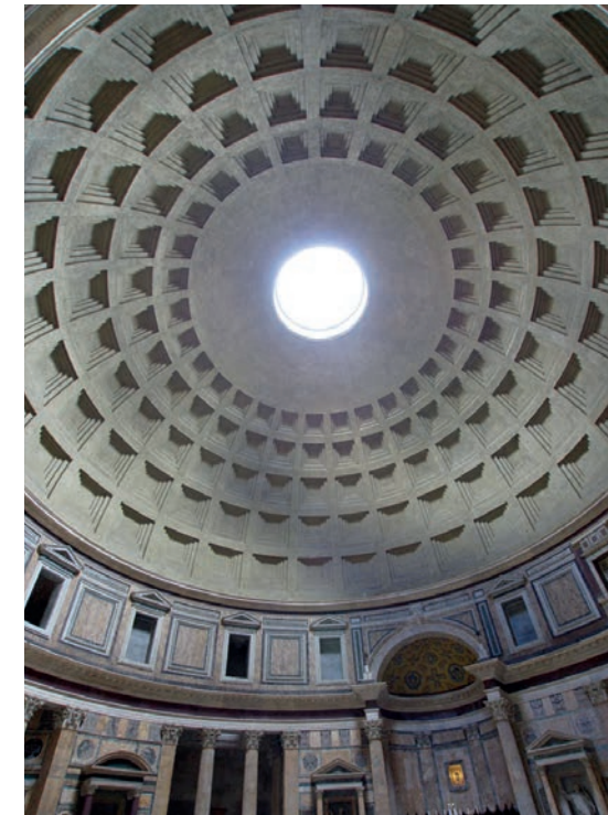
The Pantheon Temple in Rome has a limecrete dome spanning over 43m that has survived nearly 2000 years
