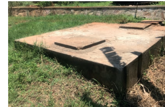
A typical underground concrete settlement chamber
