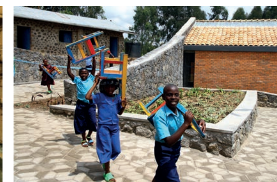
Ruhehe Primary The cement floor tiles contain volcanic stone dust as aggregate to reduce costly sand and gravel content
