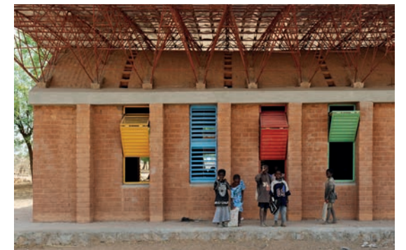
Gando School by Kéré Architecture has a barrel vaulted brick ceiling shaded by a secondary oversailing metal roof
