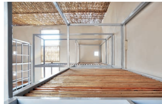
RLS Dormitory Each bed space in each of the dormitory rooms is equipped with its own personal glass block window
