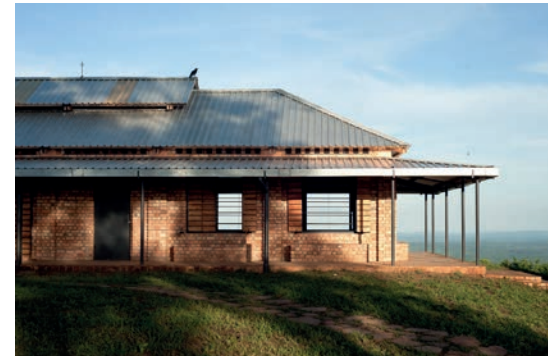
COF Primaries enjoy good cross ventilation due to shallow building depths and generous evenly spaced window openings
