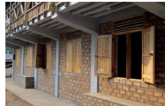
Lake Bunyonyi Secondary Windows are fitted with wooden shutters that can be open or closed to control the quantity of light
