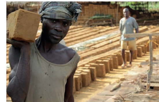
Ilima Primary Research was undertaken into using palm oil and ant-hill clay to strengthen traditional adobe mudbricks
