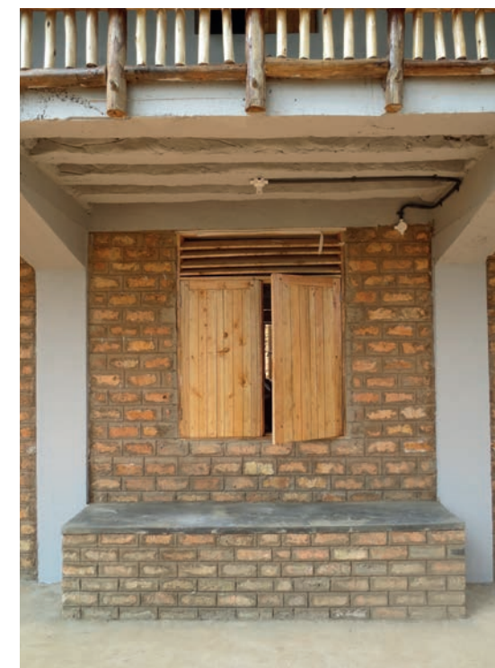
Lake Bunyonyi Secondary Classrooms have wooden shutters instead of glazing that can be manually pushed open or closed
