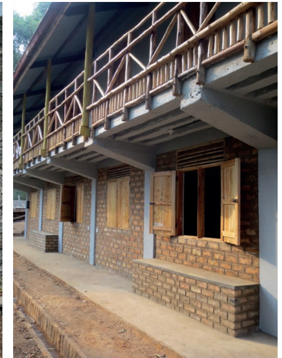
Lake Bunyonyi Secondary The boys dormitory building is an atypical 2-storey concrete structure
