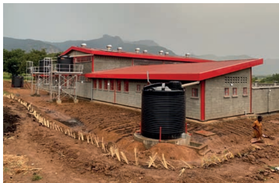
Nakapiririt VI The new workshop is provided with four PVC water tanks to harvest water from the building
