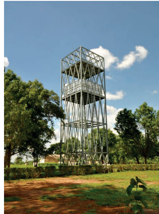
NTC Kaliro A new steel tower structure houses an 100,000L steel water tank supplied by an on-site borehole
