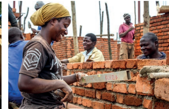
Rugerero Health Centre ASA requested a minimum 50% women workforce for construction
