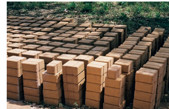
Mzuzu Health Centre Phase 1 uses a mechanical hydraform press to produce interlocking stabilised soil blocks
