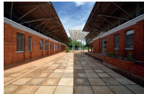
NTC Kaliro Large overhangs shade the external walls, reducing solar gain from heating the fired brick walls
