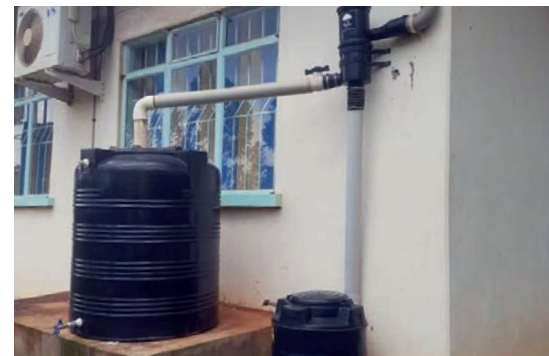
This rain filter diverts foul water through the down pipe using centrifugal force and filters clean water through a stainless steel screen
