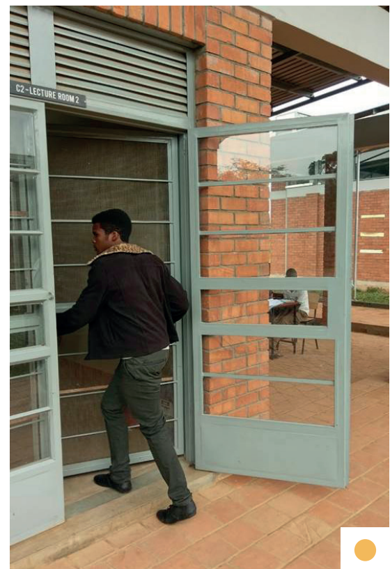
DOUBLE DOOR CONCEPT TO FACILITATE NIGHT-FLUSHING
