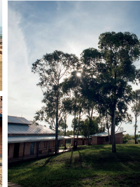
COF Primaries Classrooms are located amongst an abundance of mature trees that provide shading and evaporative cooling
