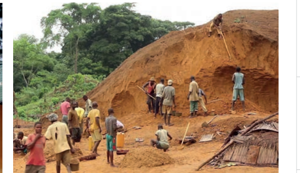
Ilima Primary Cement-free mudbricks were made with earth from nearby termite mounds to create a stronger cohesion
