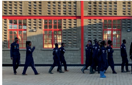
Nakapiripirit VI Thousands of louvred blocks create a large surface area of permanent ventilation openings
