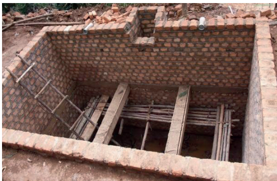
Lake Bunyonyi Secondary Temporary latrines have been replaced with two permanent four-stance latrine blocks
