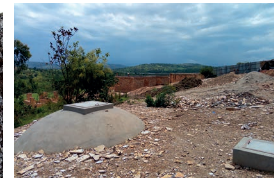
COF Primaries Toilets have an integrated biodigester that supplies the school kitchen with free cooking gas
