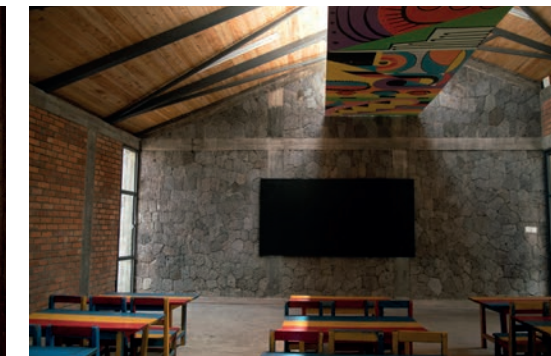
Ruhehe Primary Vibrantly decorated light shelves are hung below the ceiling to bounce diffuse light around the classroom
