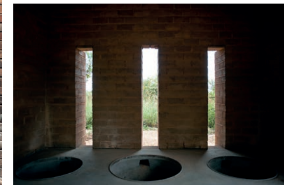
AWF Primaries The eco-stoves are fuelled with biogas supplied through a locally-made cast iron hob
