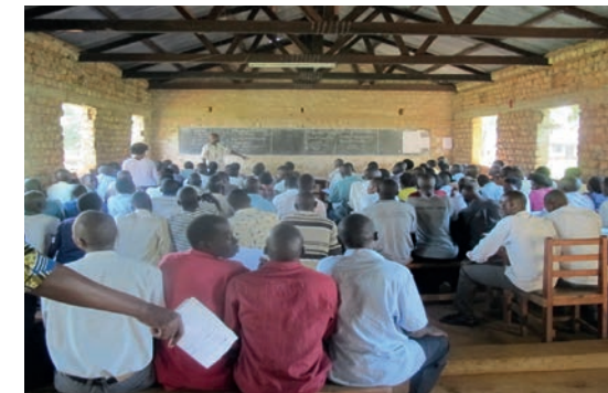
NTC Kaliro Before being renovated and expanded the NTC Kaliro had metal sheet roofing that regularly heated to over 50C
