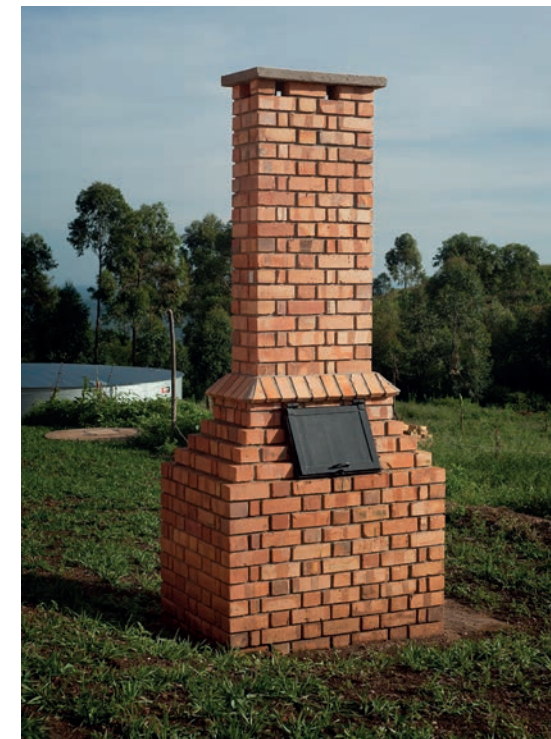
COF Primaries An incinerator is located next to the toilet block to deal with potentially hazardous sanitary waste
